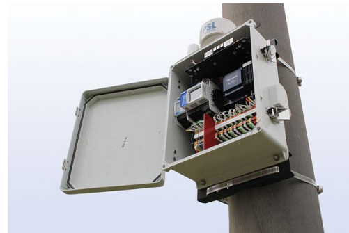
micro-PMU: Phasor Measurement Unit (PMU) for distribution applications
